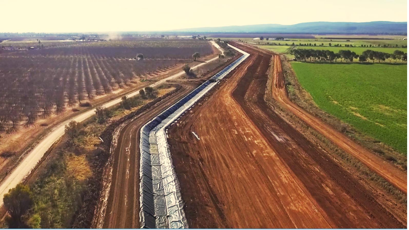
Photo: Expansion works on the Northern Branch Canal
