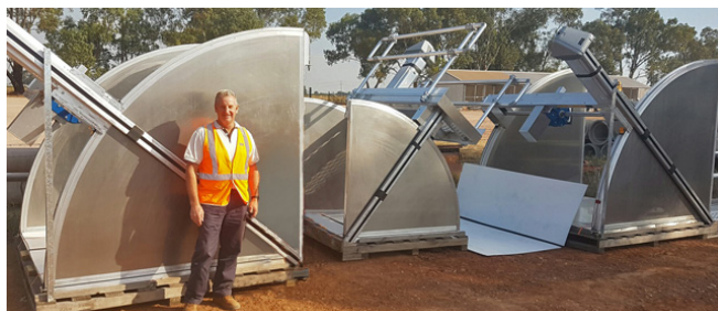
Over 90 regulator gates will be installed during the winter works program.
