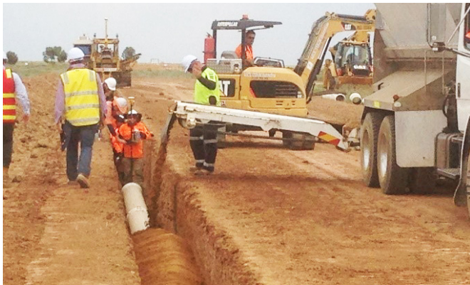
Photo: PVC pipe laying at the Main Pump Station site
