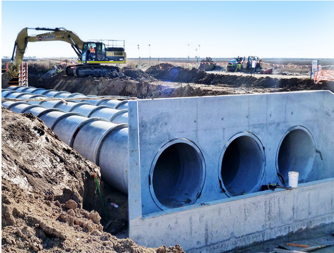
Photo: Capacity increase works, Drew Road.
