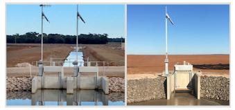
Used around our network to measure flows at regulating structures and for large (custom) on farm meters. The Slipmeter uses an ultrasonic array to measure instantaneous flow.
