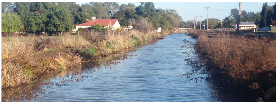
Photo: The channels in Yanco village are scheduled for rehabilitation works.
