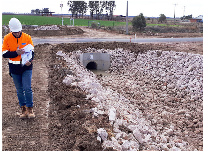
Photo: Capacity increase works, Brogden Road.
