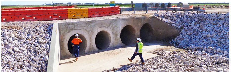
Photo: Capacity increase works, Brown Road.
