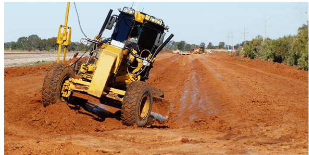
Photo: Earth channel rehabilitation works, Leeton.
