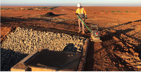
Photo: Automated outlet installation, Wah Wah.
