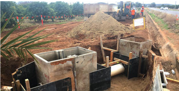
Photo: Farm outlet modernisation, Hanwood.
