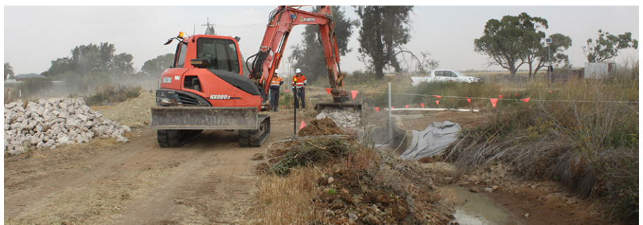
Photo: South-West Modernisation works are continuing
