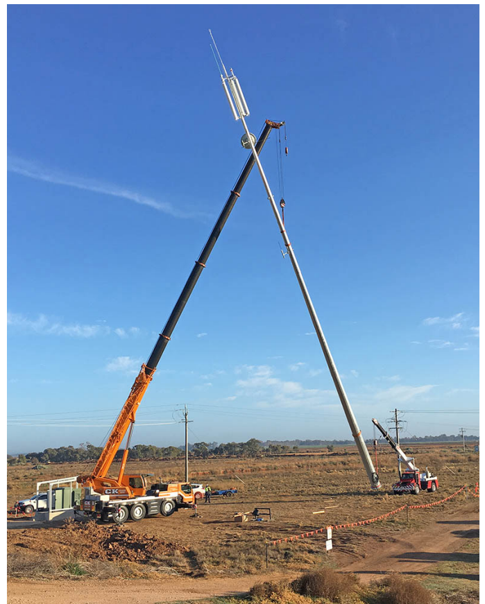
Getting connected: A Radio tower being installed.
