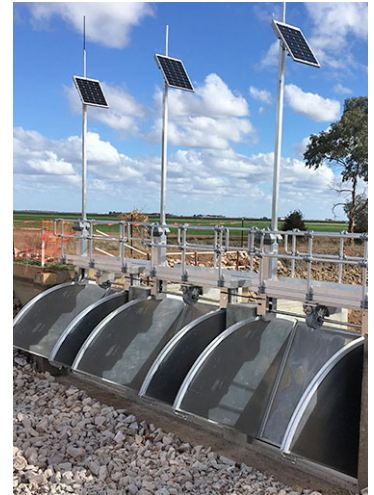
Above: Sturt Canal regulators before commissioning
