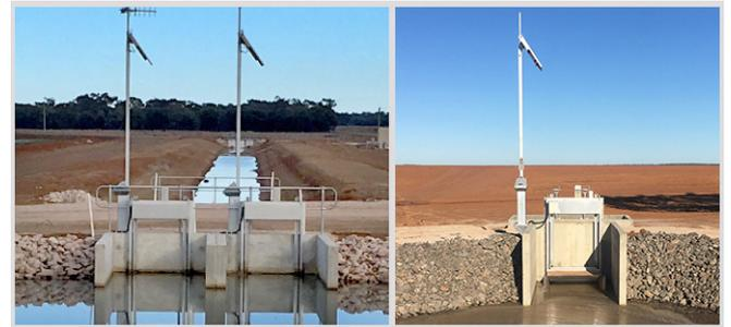
Used around our network to measure flows at regulating structures and for large (custom) on farm meters. The Slipmeter uses an ultrasonic array to measure instantaneous flow.
