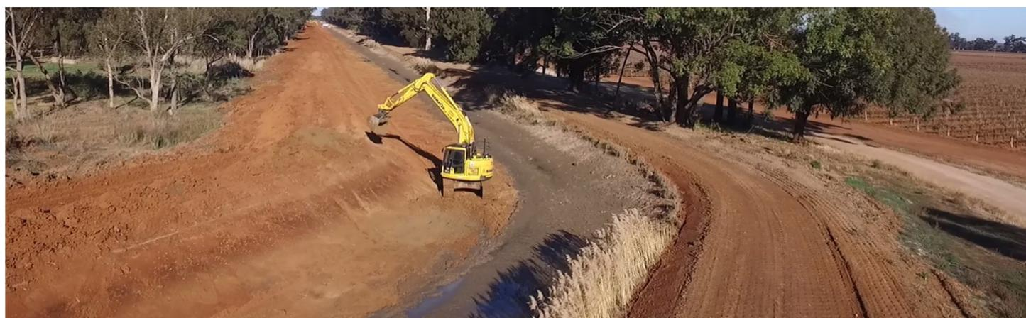
Expanding our channels and providing options around outlet sizing means we are able to deliver more water at higher flow rates, helping to grow the value of agricultural production in the region. During modernisation works in 2017, we widened 22km of the Northern Branch Canal to effectively double its capacity. Working in partnership with our NBC customers has allowed us to deliver more water and higher flow rates to meet their changing needs and build a better network for the future.
