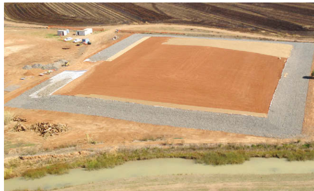
The Contaminated Land Remediation Project involved the containment of large amounts of illegally dumped asbestos within an earthen mound.
