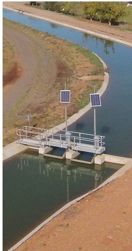
Automated channel regulators in the Lake View Branch Canal regulate water levels for timely water deliveries and increased system efficiency.
