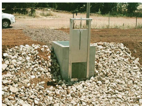
One of several outlet replacements at Murrumbidgee.
