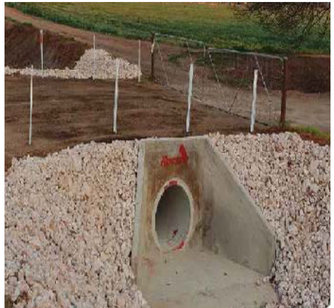
A culvert providing access to a customer's property.
