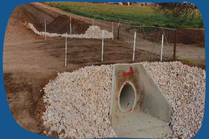
A culvert providing access to a customer's property.
