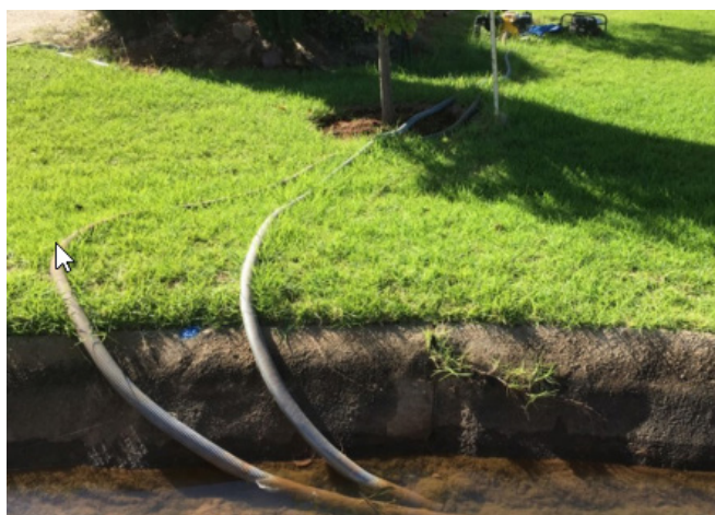
An example of unauthorised access
