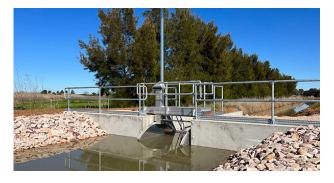
Our 2022 winter works program included the automation of 140 outlets and 80 regulators in Murrami and Yenda, as well as the lining of 4 kilometres of channels, as part of our ongoing Automation Project.
