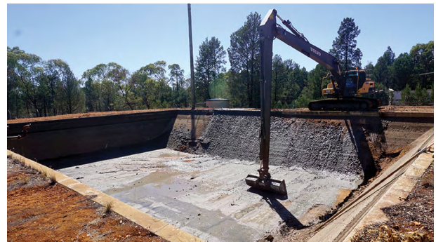
MI equipment cleaning dam at the top of Scenic Hill, Griffith
