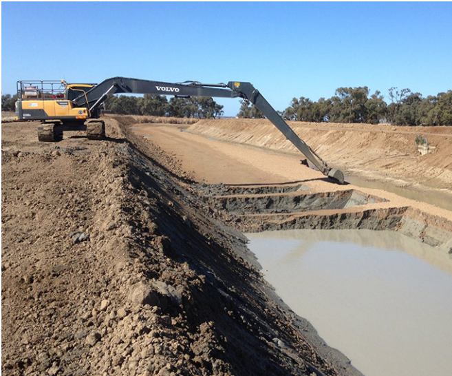
Extensive desilting works on the Sturt Canal
