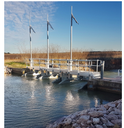
Automated regulator, Sturt Canal
